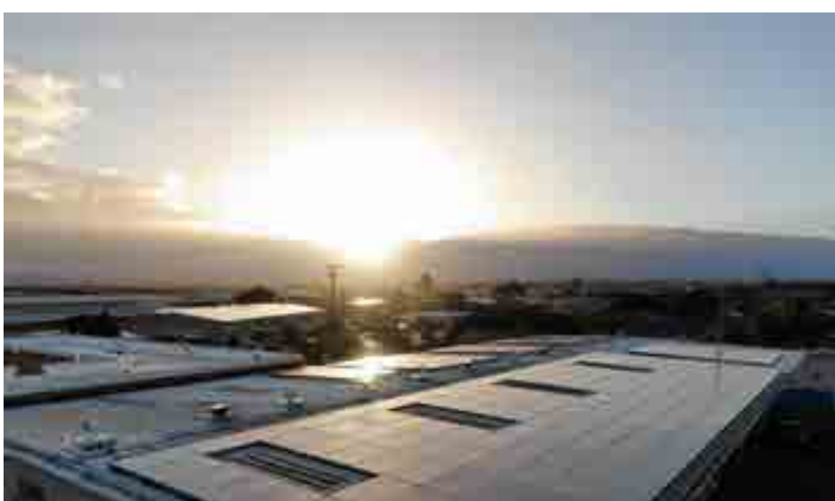
Shared solar project on a business in Kahului, Maui. This 28-kilowatt project came online in 2021.
